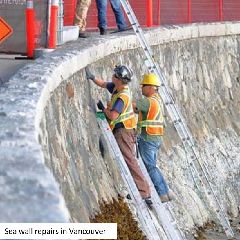
Ecological niches created through texturizing wet cement
