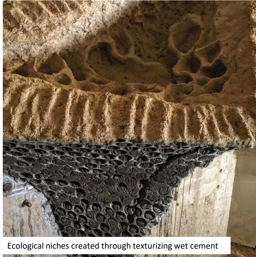
Small scale patching
